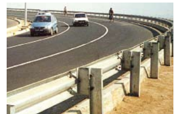
Road Safety Systems
